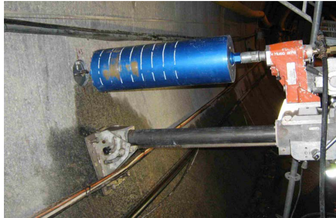
Figure 3. The LVDT-probe installed in a pilot hole and ready for overcoring.
